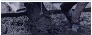
**12. Surface Tolerances (Based on ACI 302, Section 8.15)** In the past, floor profile quality had been specified by limiting the size of the gap measured under a 10 ft. (3 m) long straightedge placed anywhere on the floor. Today, the Face Floor Profile, or "F-number" system provides a more accurate method for specifying, executing, and measuring the surface tolerance of a floor.
