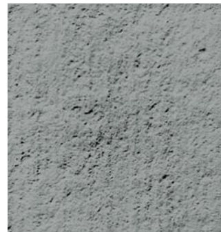
CSP 4 (light scarification)
